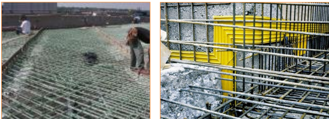
Figure 20: Rebar and Water Bar Installation
